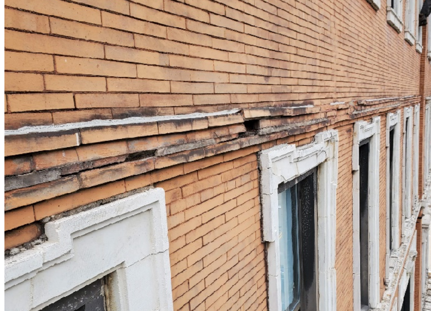
Brick repair at floor line
