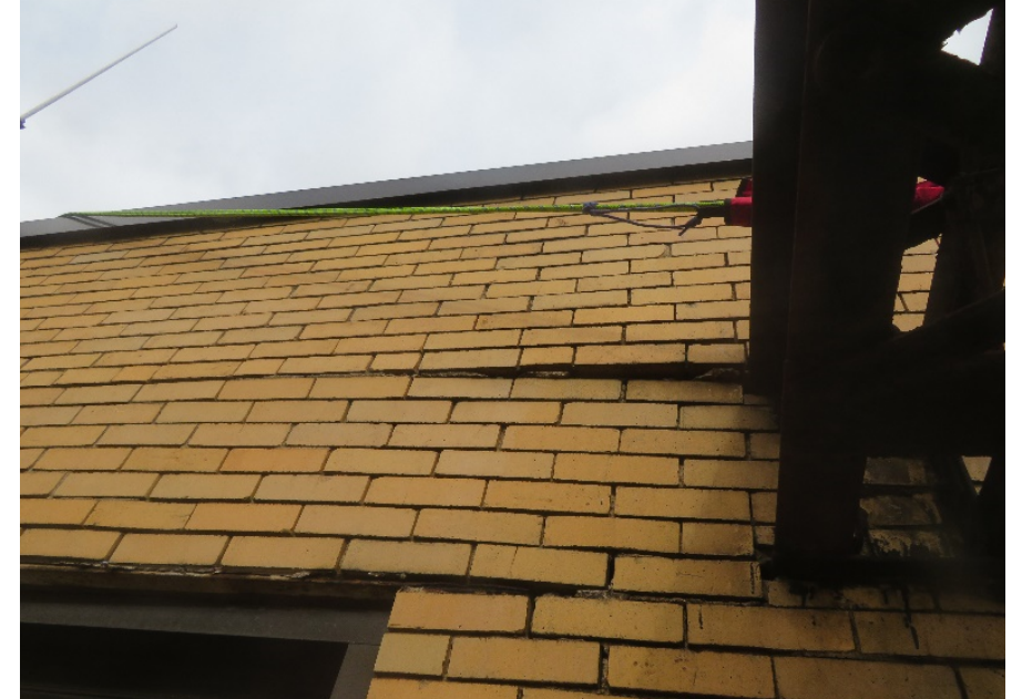
Movement at parapet
