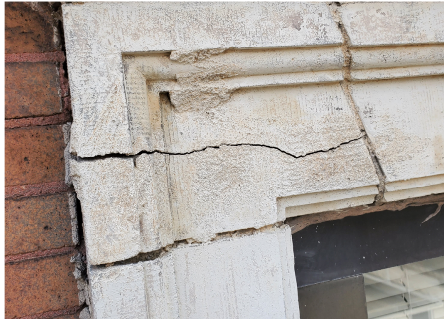
Cracking at lintels
