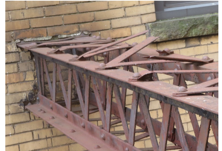
Corrosion at exterior beam
