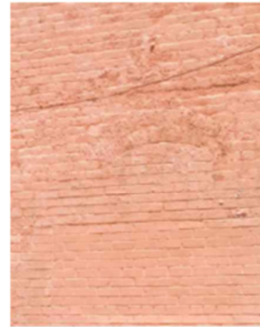
Brick is already painted. Point and repaint.
