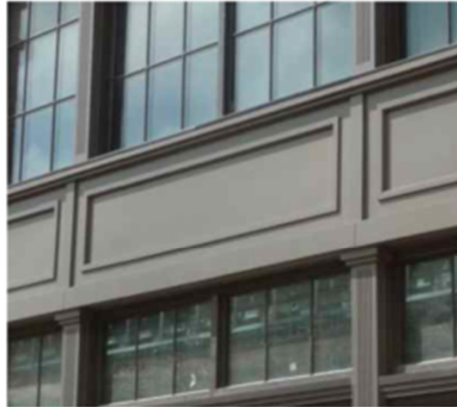
PVC millwork for below storefront, casings, cornice detail above storefront, soffit/fascia. Field painted.
