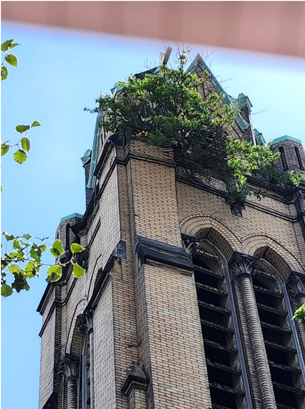
Photo No.2 –Bell Tower. Note vegetation and loose & damaged masonry.
