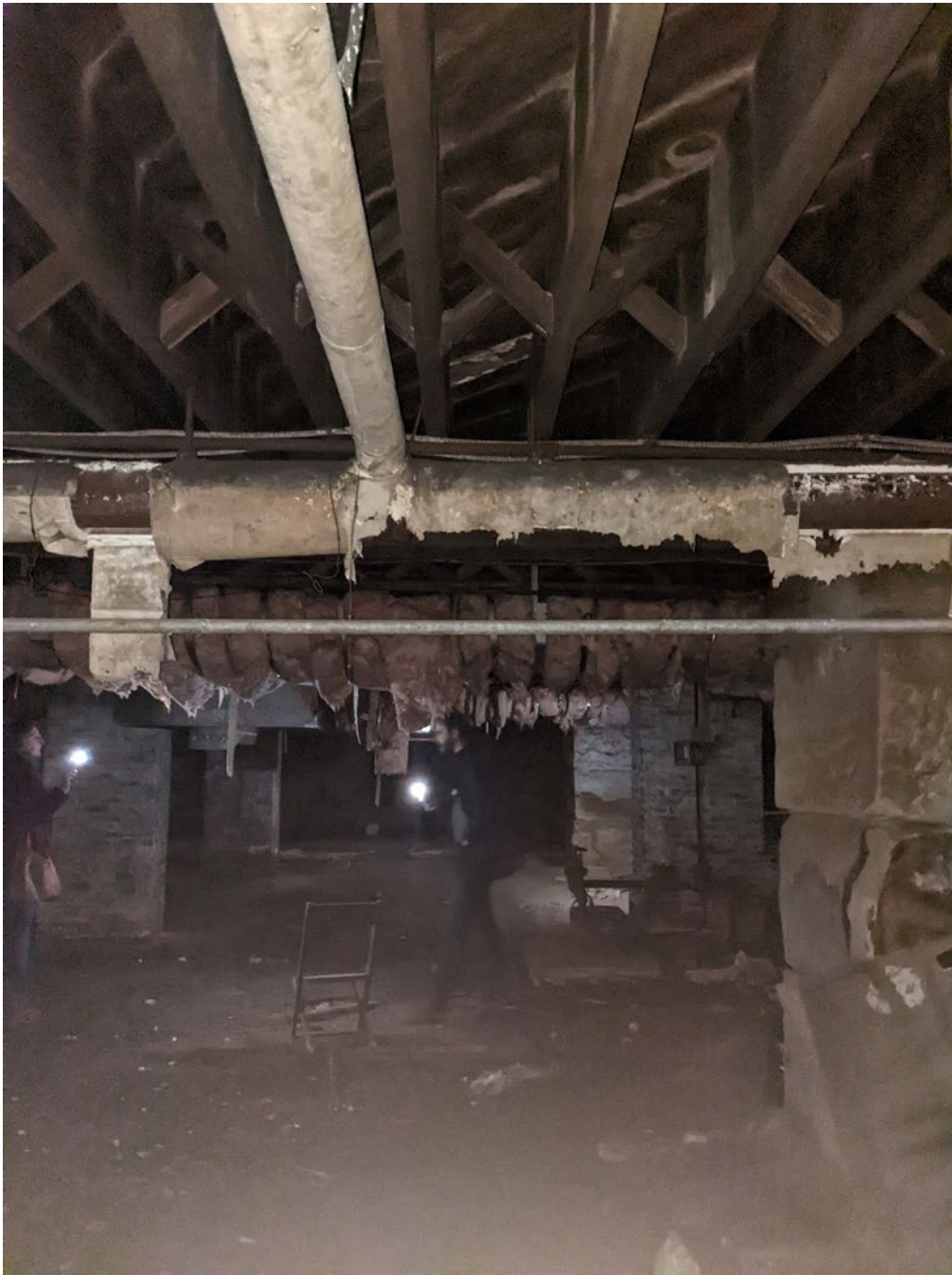
Photo No.6 –View of first floor framing from basement, note stone and brick masonry piers in background and exposed ground floor.
