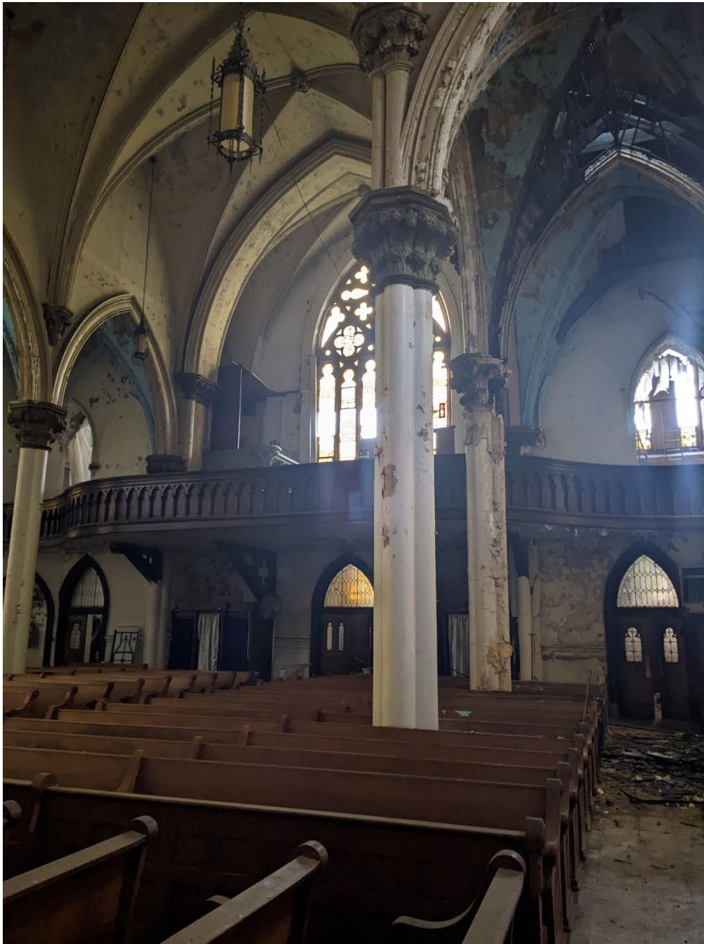
Photo No.11 –View of first floor looking toward the rear of the nave (looking southwest toward Liverpool). Note the failed roof condition and deteriorated condition of the adjacent wall construction and the missing stained glass beyond.
