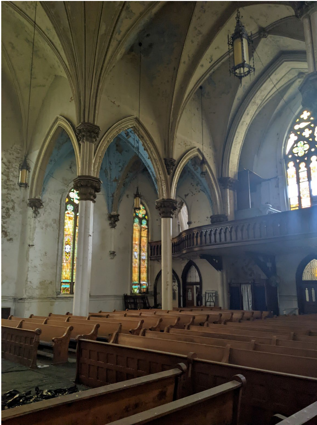
Photo No.12 –View of first floor looking toward the rear of the nave (looking southeast). Note the failed roof condition and deteriorated condition of the adjacent wall construction and the missing stained glass beyond.
