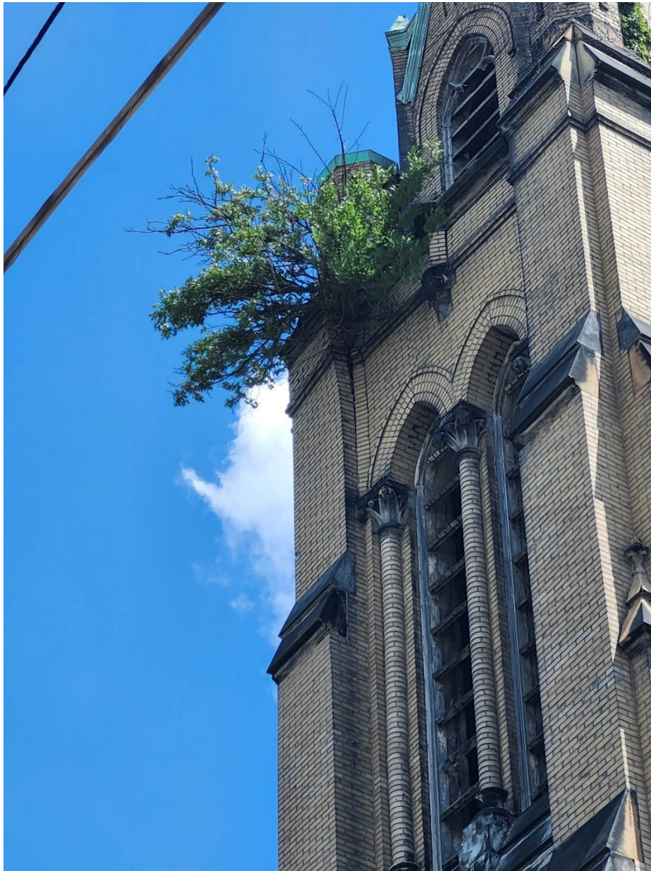
Photo No.4 –Bell Tower. Note vegetation and loose & damaged masonry.
