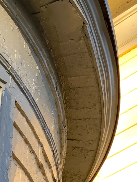
Paint shadows under soffit of south bay window, showing spacing, depth and width of former dentils.
