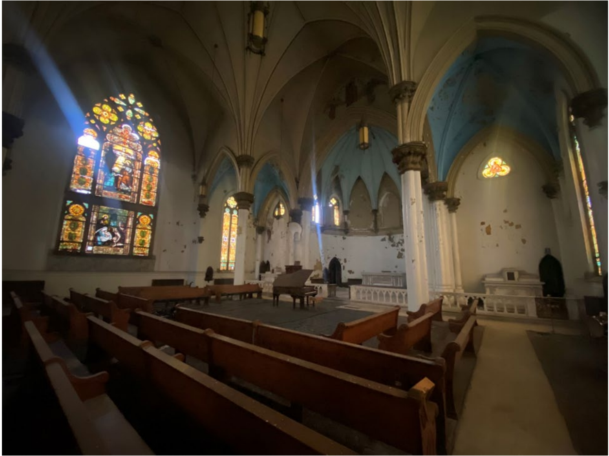
Photo No.7 –View of first floor looking toward the chancel. Note missing stained glass in window, peeling paint and plaster on walls and ceiling.
