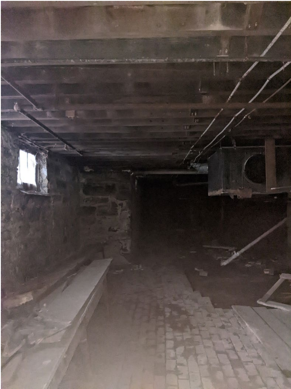
Photo No.5 –View of stone masonry basement wall and wood block flooring.
