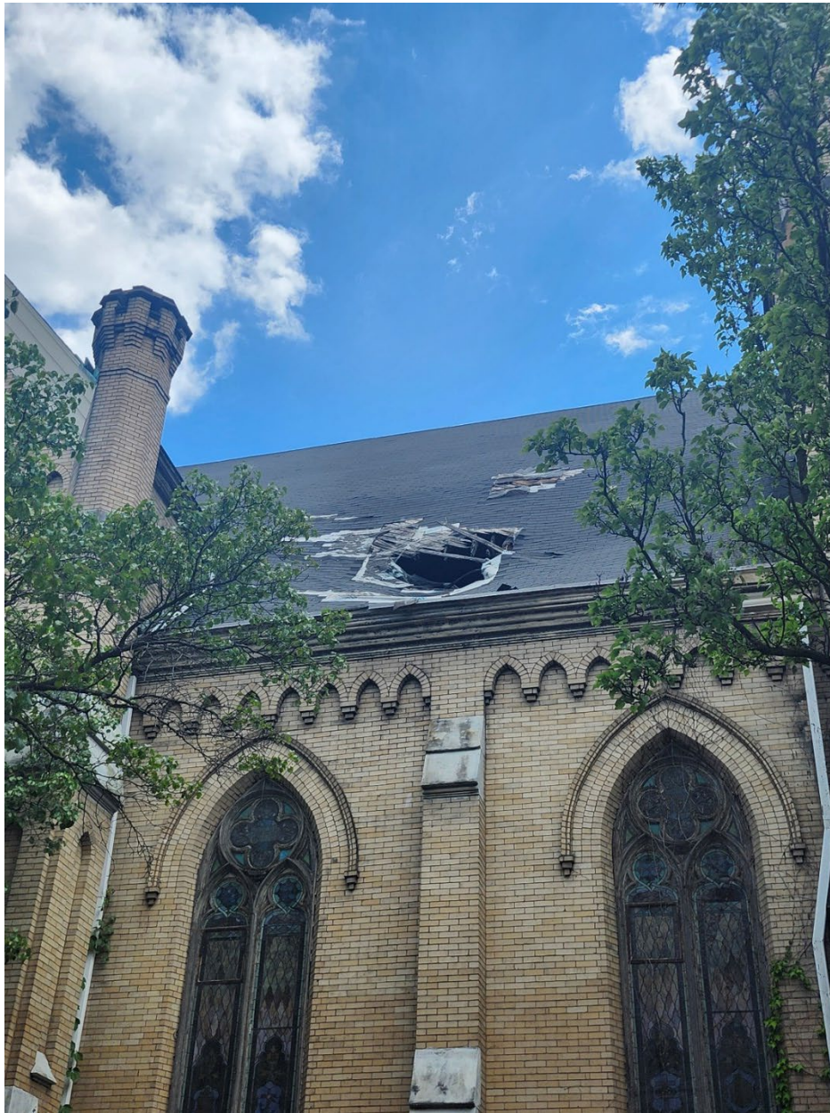
Photo No.14 –Exterior view of roof failure above the nave on the west side of the building (along Decatur).
