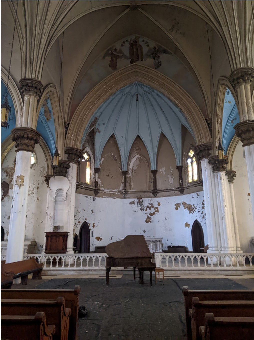
Photo No.9 –View of first floor looking toward the chancel and aspe. Note the peeling paint and plaster and damaged and missing stained glass in the windows.
