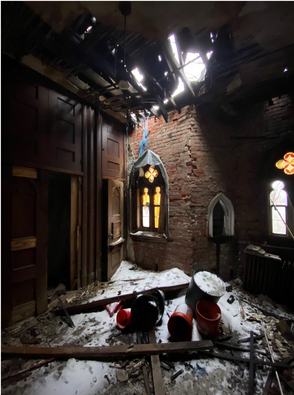
Photo No.13 –Interior view of roof collapse above the chapel at the northwest corner of the building.
