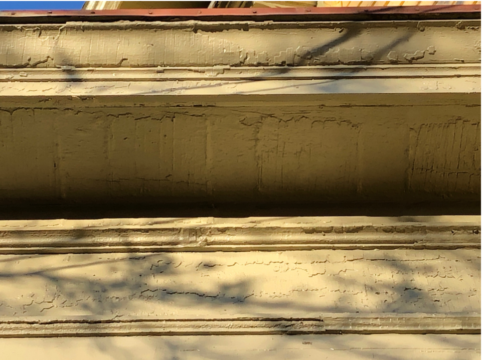
Paint shadows under soffit of west bay window, showing spacing, depth and width of former dentils.
