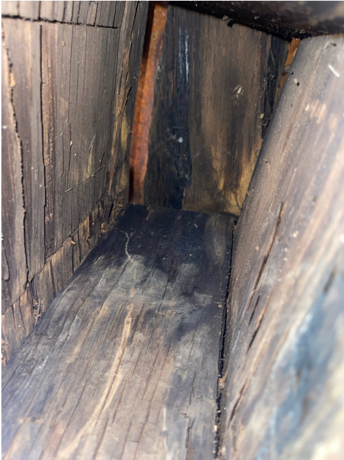
Original porch box beam. Original porch structure will be retained and repaired where possible.
