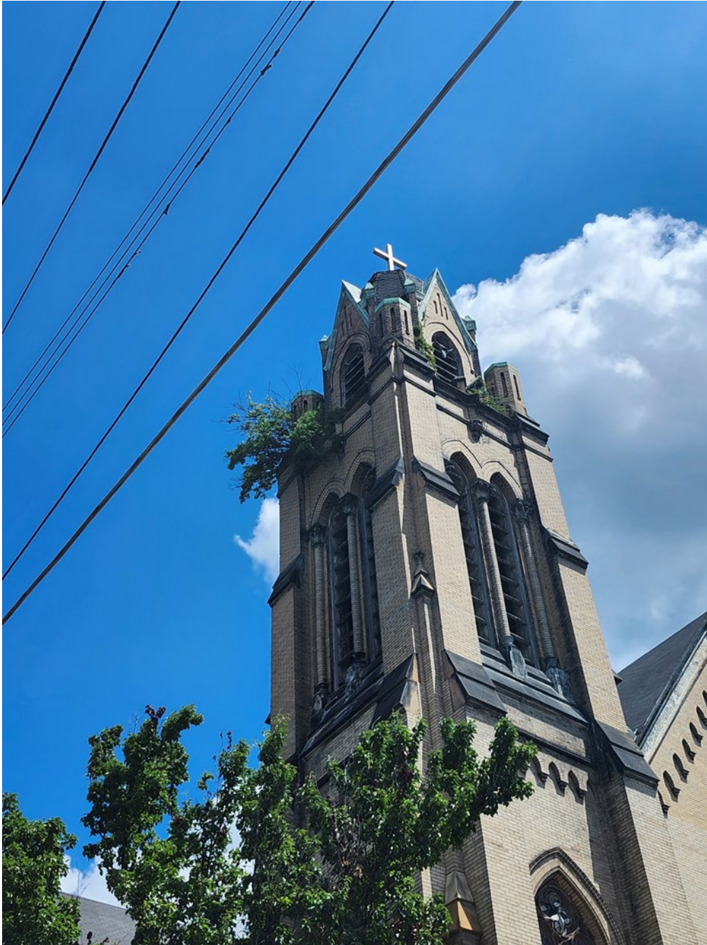
Photo No.3 –Bell Tower. Note vegetation and loose & damaged masonry.
