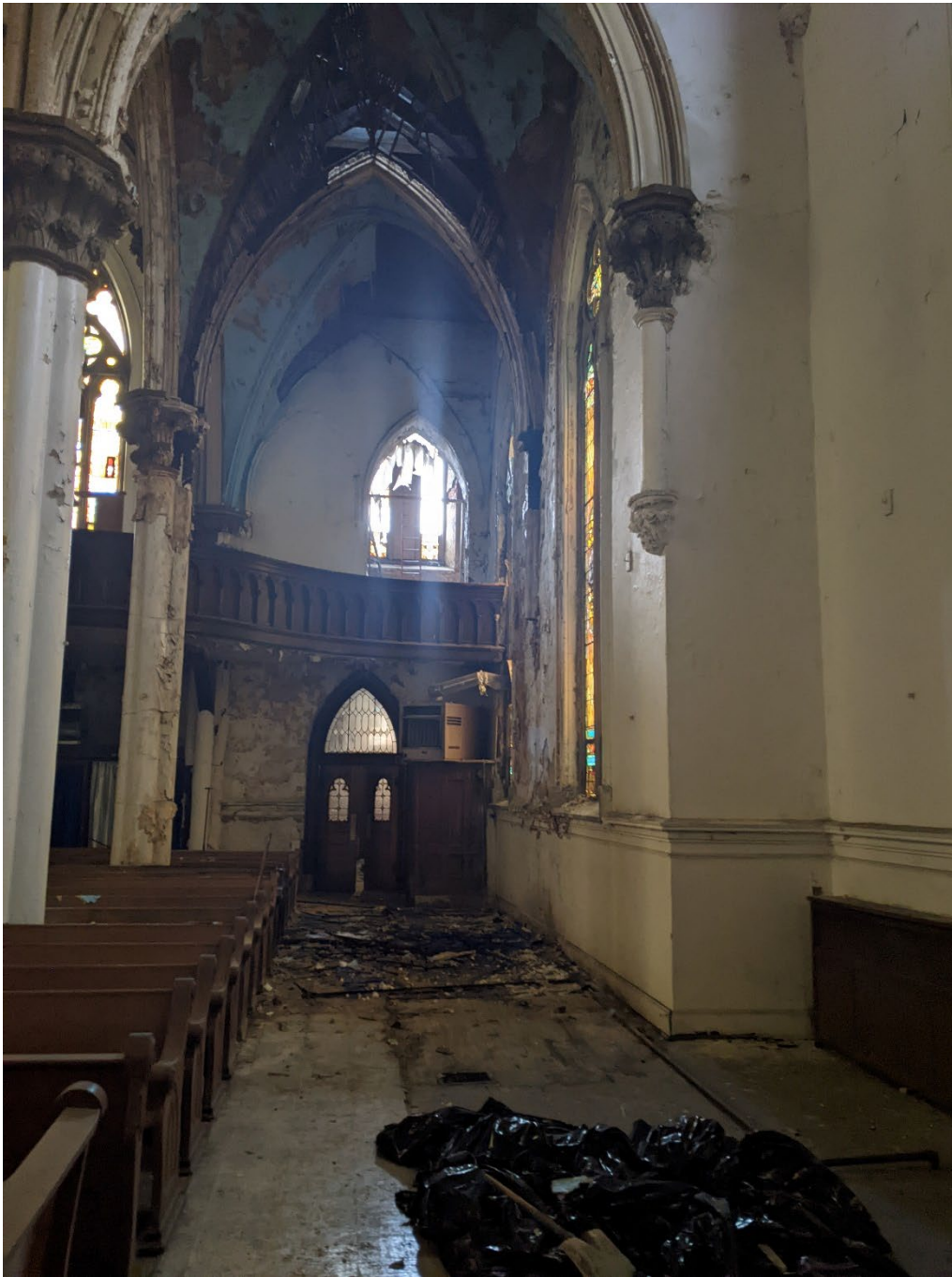
Photo No.10 –View of first floor looking toward the rear of the nave (looking southwest toward Liverpool). Note the failed roof condition and deteriorated condition of the adjacent wall construction and the missing stained glass beyond.
