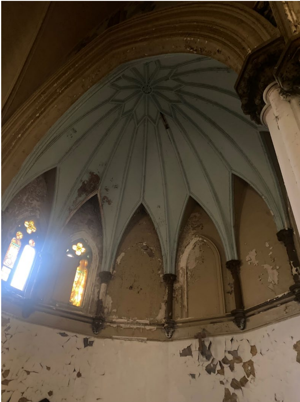
Photo No.8 –View of first floor looking toward the dome above the aspe. Note the peeling paint and plaster and damaged and missing stained glass in the windows.
