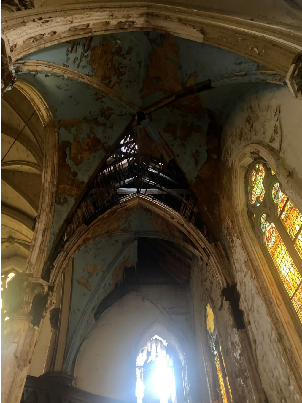
Photo No.15 –Interior view of roof failure above the nave on the west side of the building (along Decatur).
