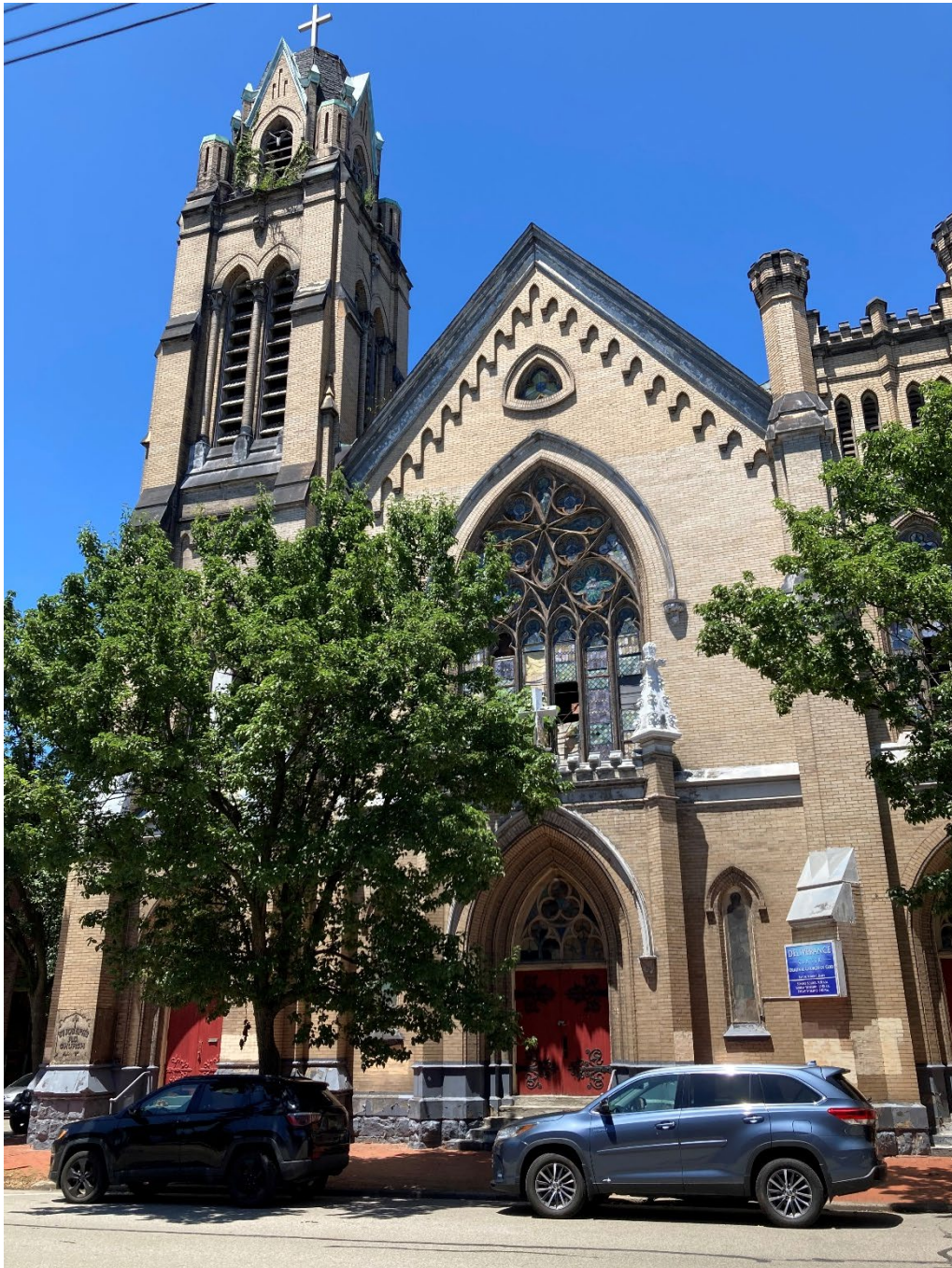
Photo No.1 –Front elevation of the Building. Note broken and missing stained glass and vegetation growing from the bell tower.
