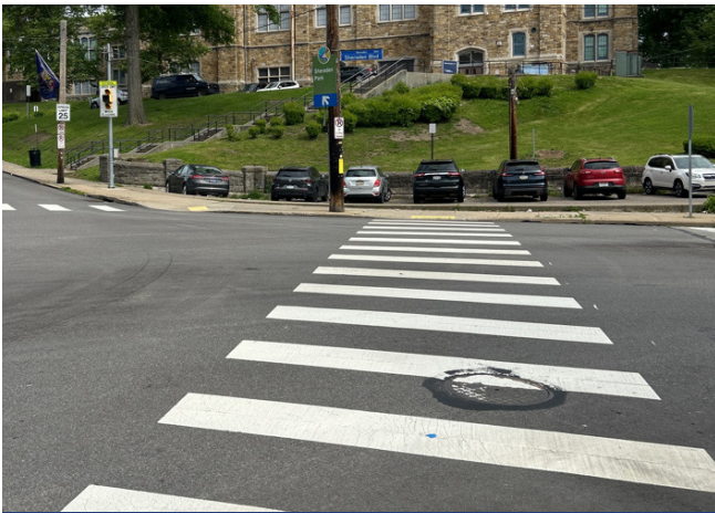
Wide intersections result in long pedestrian crossings, such as this one in front of Langley Elementary.
