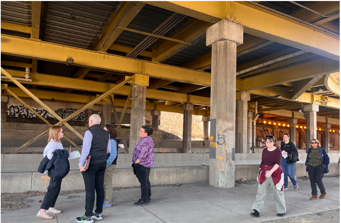
FIGURE 19 Stakeholders walk under the West End Bridge at West Carson Street - Highways, topography, railroads, and rivers are barriers to mobility throughout West Pittsburgh.
