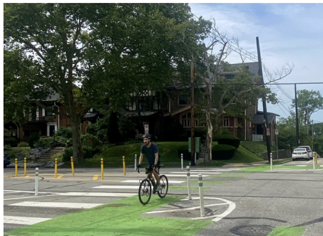
FIGURE 31 The City of Pittsburgh regularly installs safety treatments throughout the city. Examples here include pedestrian refuge island, speed table, traffic diverter, and painted curb extensions for transit riders. (courtesy of the City of Pittsburgh)
