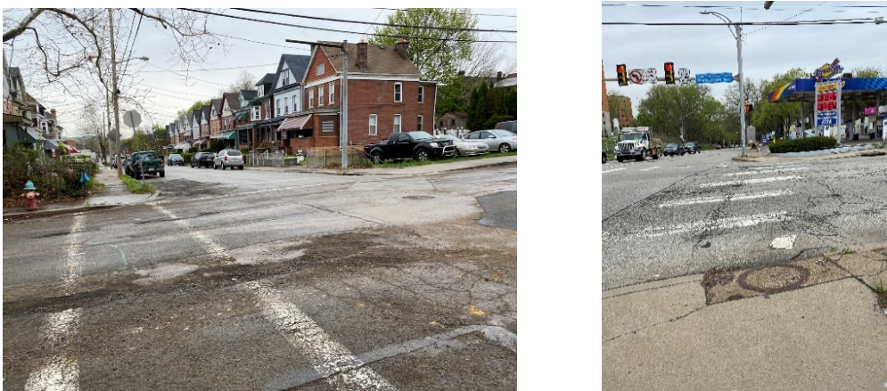
Figure 8: Faded Pavement Markings in Homewood
