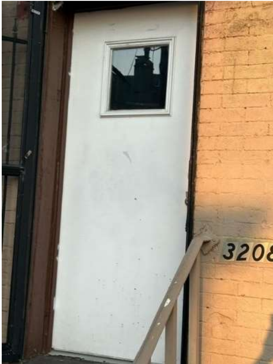
3. Front door on 1 st floor facing street: Main entrance of Unit1
