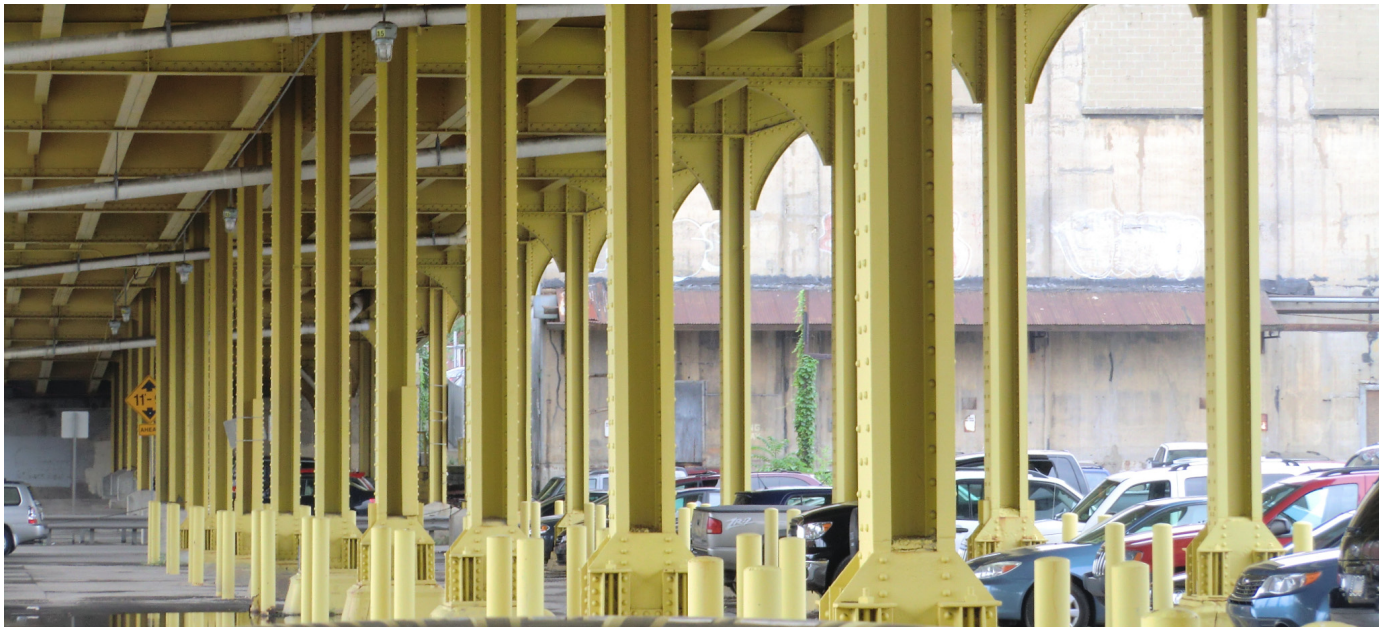
23 16th Street Bridge Underpass
