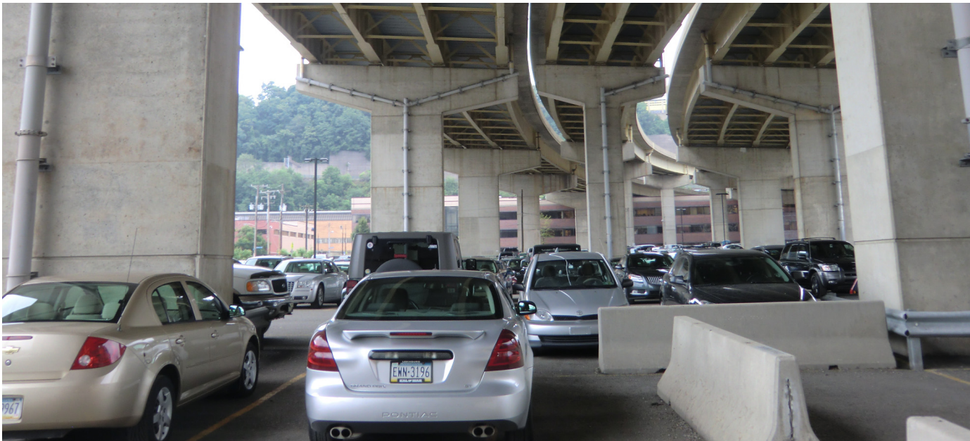
22 Veterans Bridge Underpass
