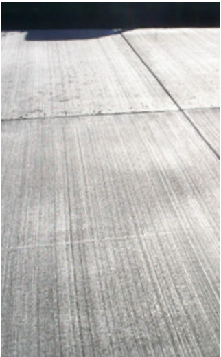
Broom Finished Concrete
