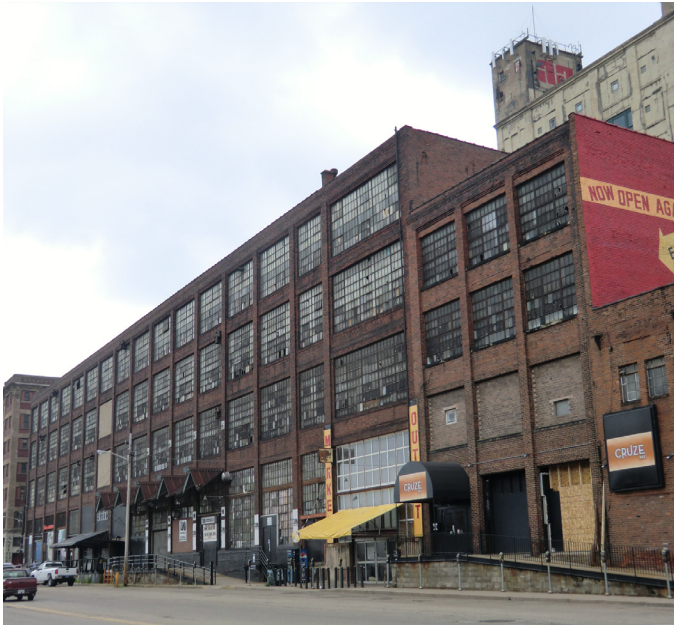
5 Warehouse Facilities Numerous former warehouses still existing in the project area. The predominant material of buildings in the area are brick and glass.
