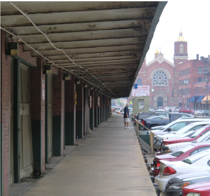
2 Loading Docks Loading docks are elevated.
