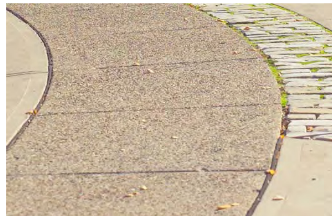
Exposed aggregate paving with Belgium block edge
