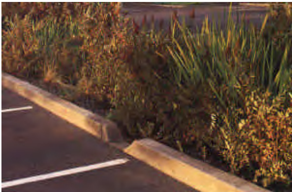
Example of bioswale
