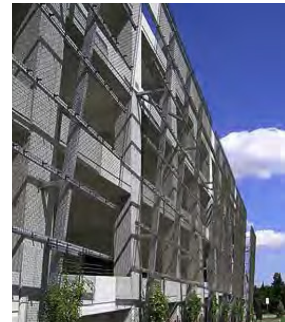
Metal screening layers a concrete garage structure.
