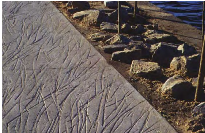
Imprinted Concrete Paving
