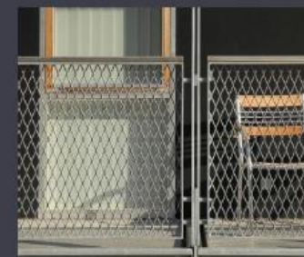
Metal Mesh Railings
