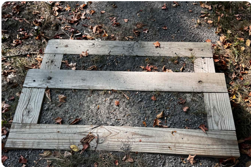
wood box steps | a proven stair method in the pittsburgh parks.
