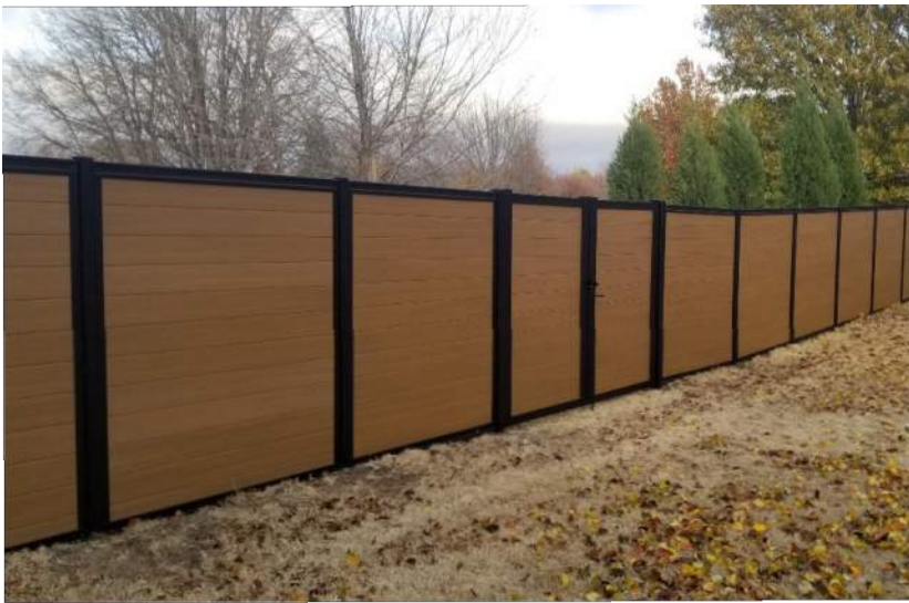
ELECTRICAL EQUIPMENT SCREENING WALL
