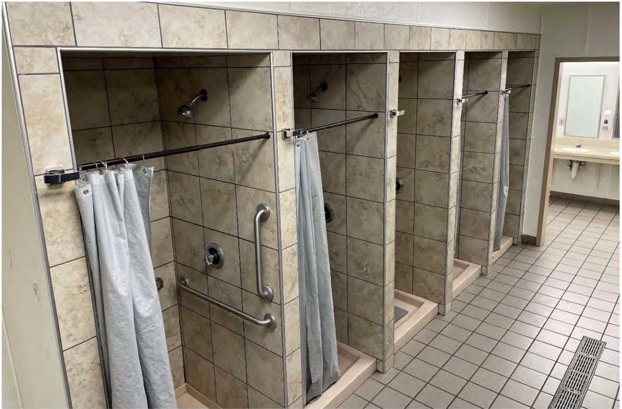
Typical Bathroom showing Handicapped Accessible Showers, Toilets & Urinal
