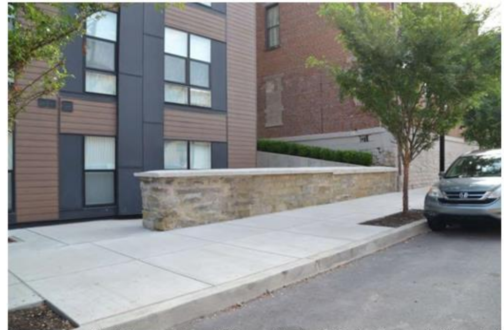
Photo 3: Stone Wall Segment along 39 th Street, North of Officer's Quarters Building, Looking Southeast
