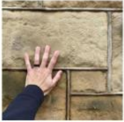
Ashlar sandstone w/ Beaded mortar Music Building
