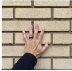
Tan brick with raked joints Ruskin Hall
