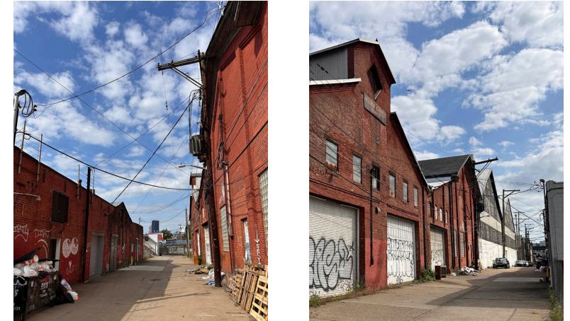
Warehouse buildings, View from Mulberry
