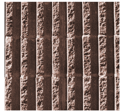
decorative block wall - ground floor
