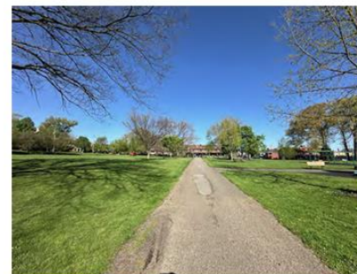
Photo 2. Westinghouse Park, Footpath looking Northwest.
