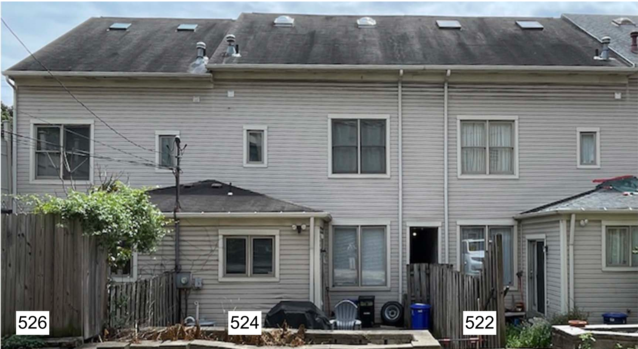
EXISTING CONDITIONS - REAR
