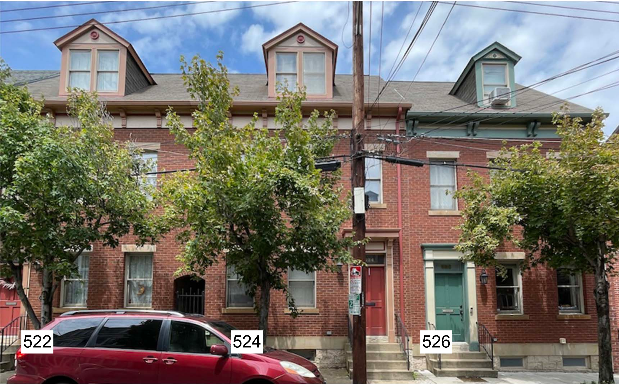
EXISTING CONDITIONS - FRONT
