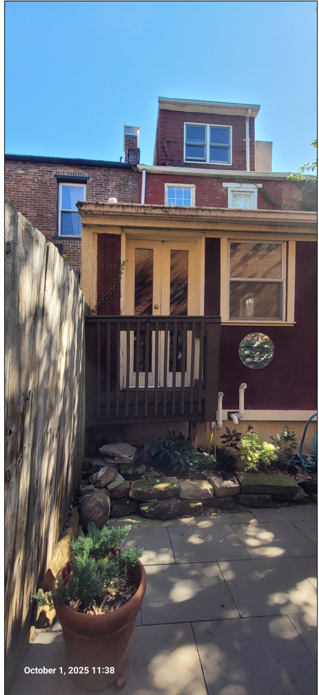
1403 Sherman Avenue Existing Rear Facade - View from Rear Yard
