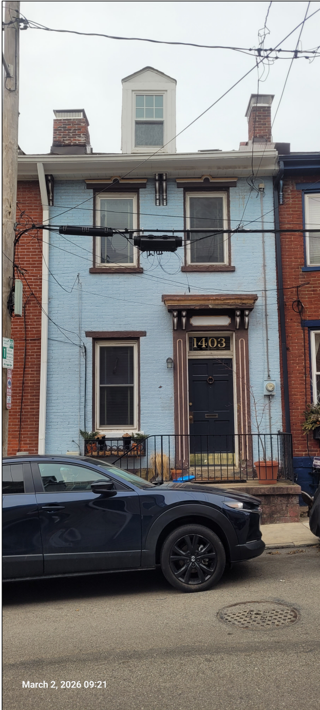
1403 Sherman Avenue - Existing Front Facade - View from Sherman Avenue
