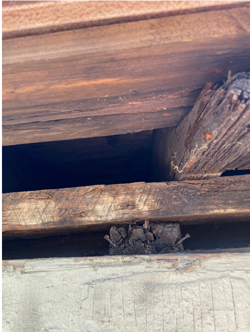
Wood outriggers will be sistered to existing porch roof when box gutter is rebuilt.
