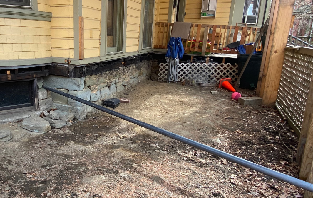
Foundation wall will be repaired and repointed w/ appropriate, Type N mortar.
