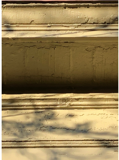
The shadows of missing porch cornice dentils are visible.
