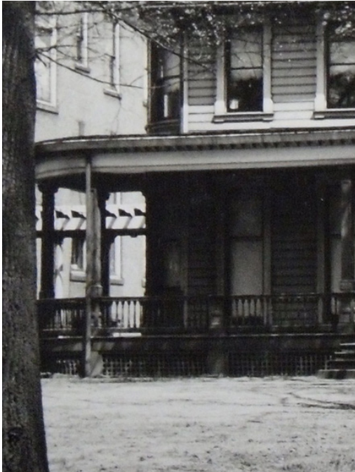
Porch cornice dentils are visible in historic photos, but they are no longer present.
