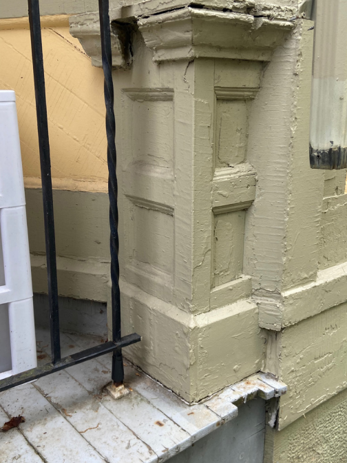
Profile of original porch top rail and base rail are visible.
