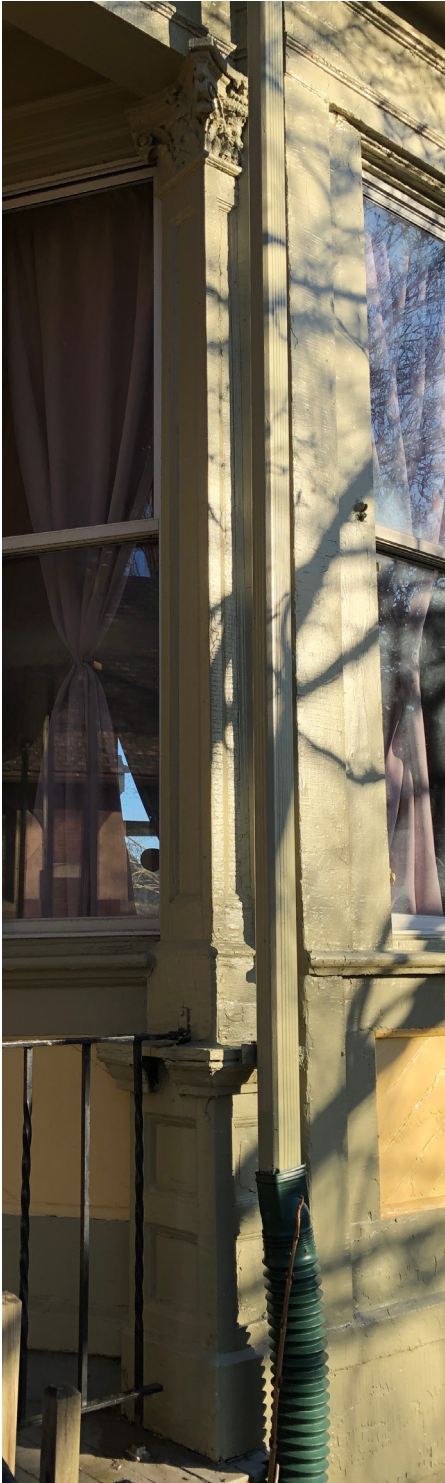
The existing, original Pilaster, including the Composite-style capital, post and base, will serve as a model for new Porch Posts and Pedestals.
