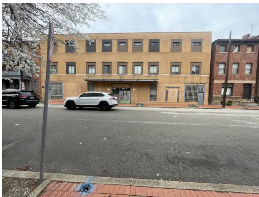
1217 Liverpool St. HRC.4: Existing Site Photos Cont.
