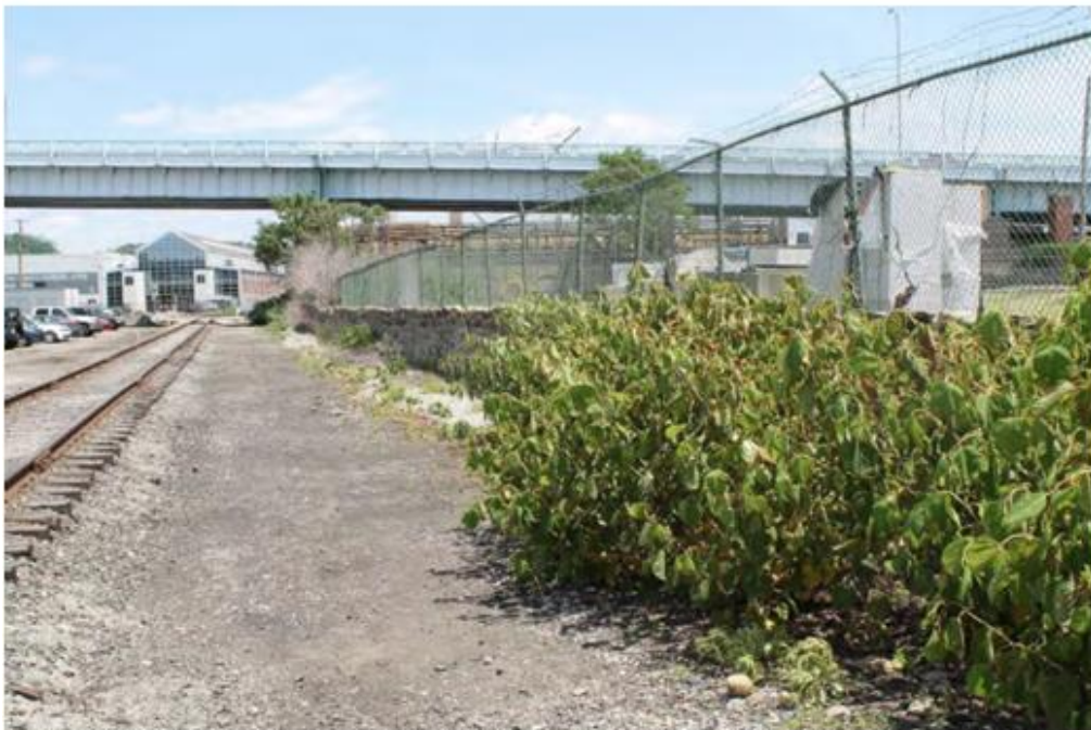
Photo 2: Stone Wall Segment, Warf Wall, Looking Northeast (May 2016)
