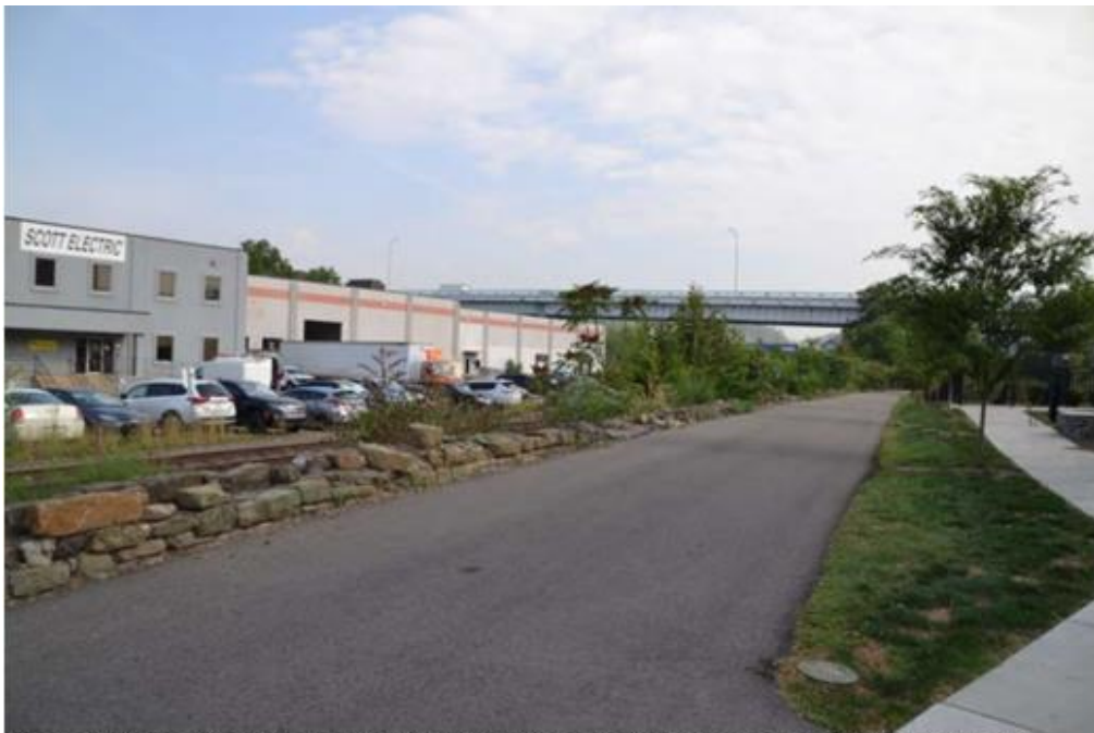
Photo 1: Stone Wall Segment, Warf Wall Along Railroad Tracks, Looking Northeast
