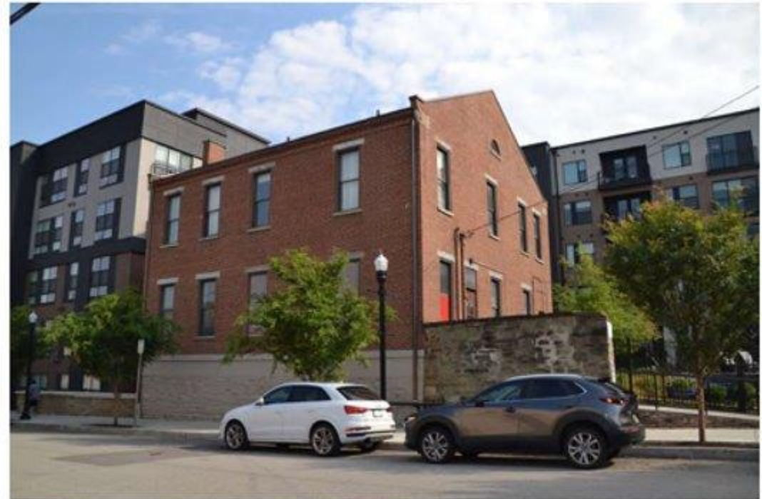
Photo 23: Southwest façade of Officers' Quarters Building, Looking North
