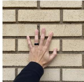
tan brick with raked joints Ruskin Hall
