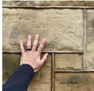
ashlar sandstone w/ beaded mortar Music Building
