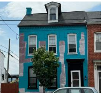
Example of inappropriate use of paint on masonry substrates, as well as inappropriate color choice.
