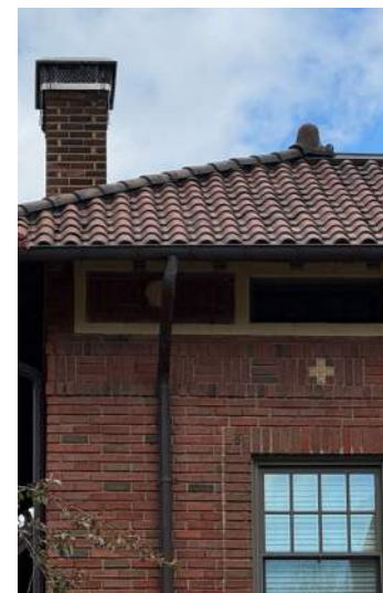
An example of a Spanish clay tile roof.
