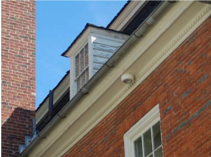
Modern facade lighting is concealed under the eve and the fixture color blends in; this is an appropriate installation.
