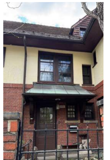
An example of a slate roof and metal entry hood.
