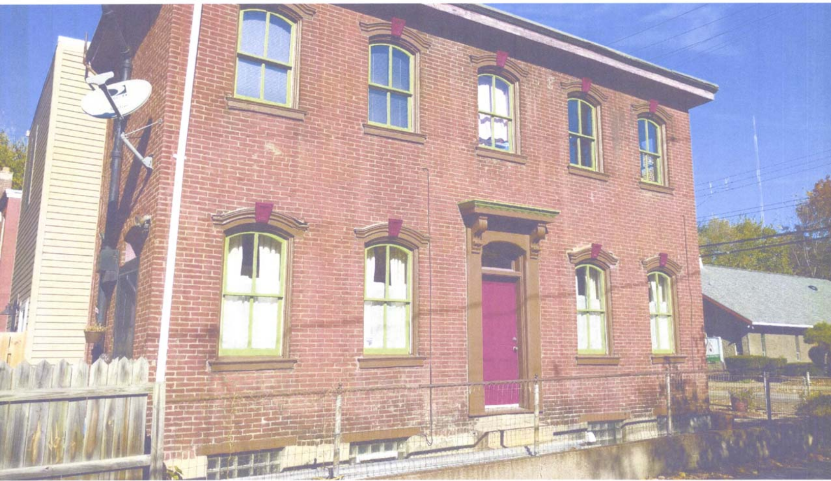
1401 BUENA VISTA ST. - SOUTH (SAMPSONIA WAY) FACADE
