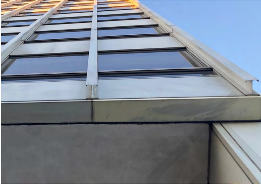
Photo 7. Facade detail showing steel I-beams applied between window bays
