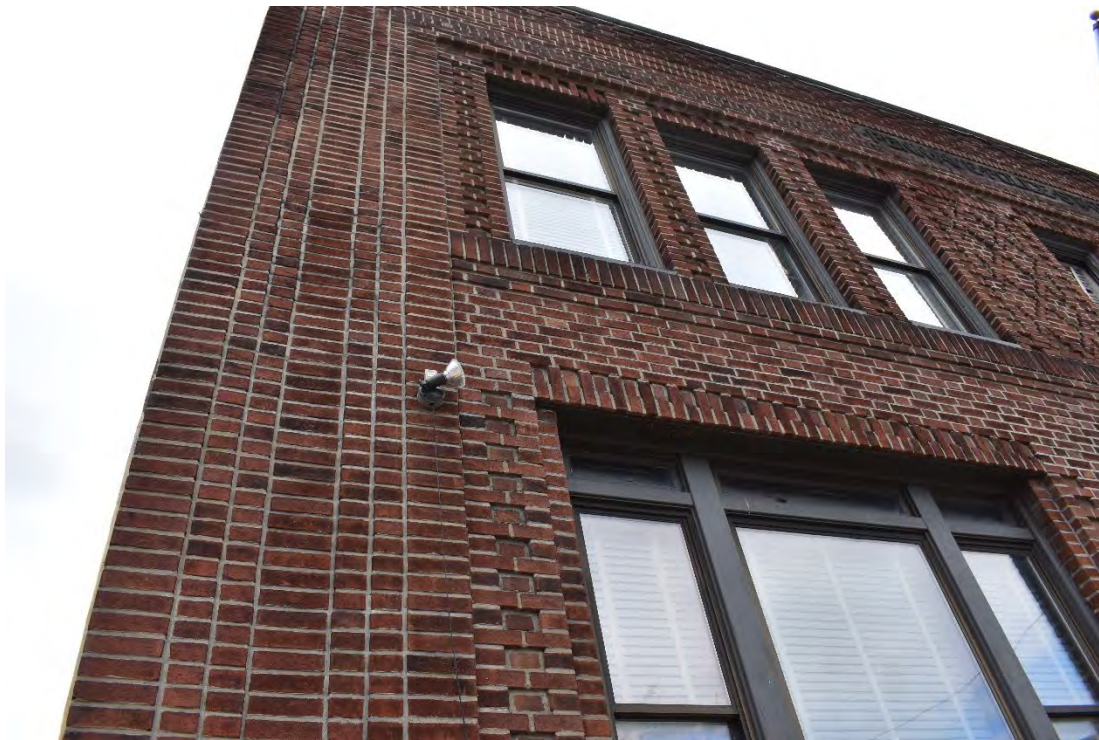
Photograph 5. View of perimeter brickwork detailing, created using bricks laid both horizontally and vertically, as well as turned end-on-end. (Amanda Stander 2020).
