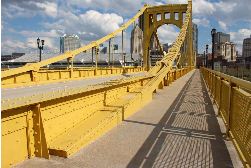
Photo 14. Rachel Carson Bridge (April 2024), detail of attachment point of west eyebar chain at northwest bridge quadrant, facing south.
