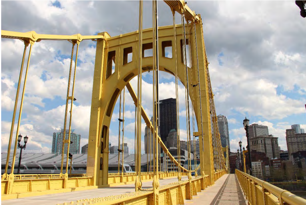
Photo 16. Rachel Carson Bridge (April 2024), overview of north tower and sidewalk side of built-up stiffening girder and lower stirrup-and-eyebars connections, facing southeast.
