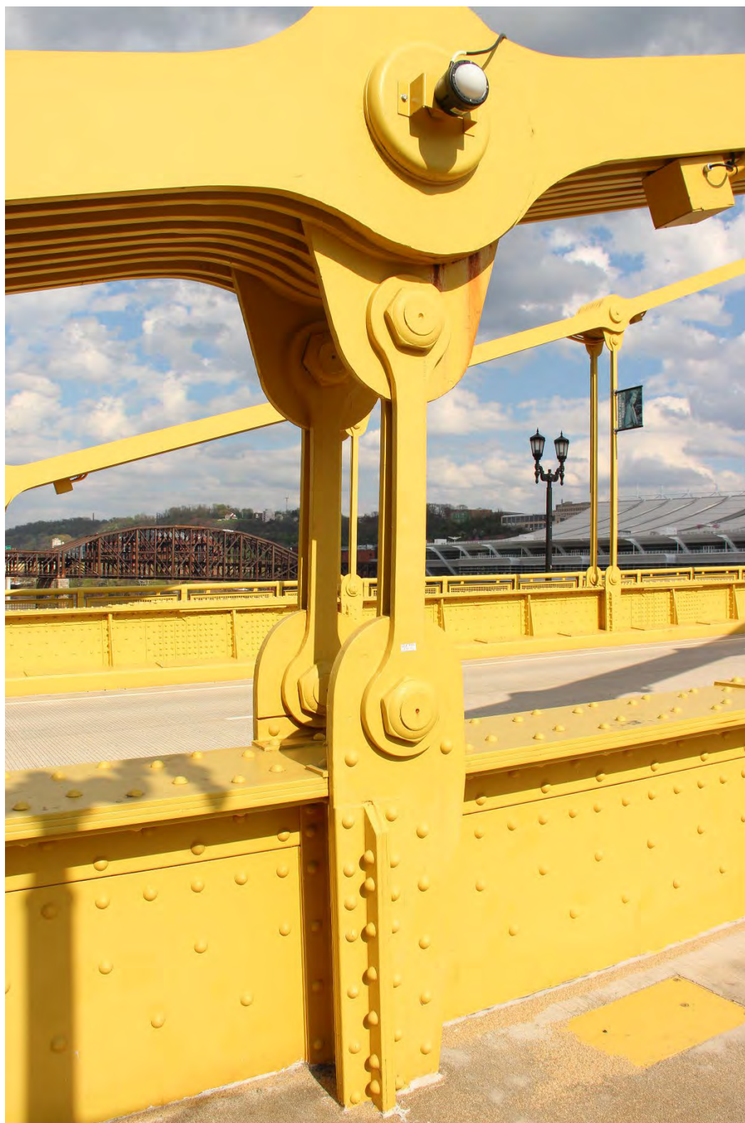
Photo 15. Rachel Carson Bridge (April 2024), detail of detail of pin-connected eyebar suspenders and stirrups in northwest part of bridge, facing southeast. An LED light is visible covering the eyebar chain pin.
