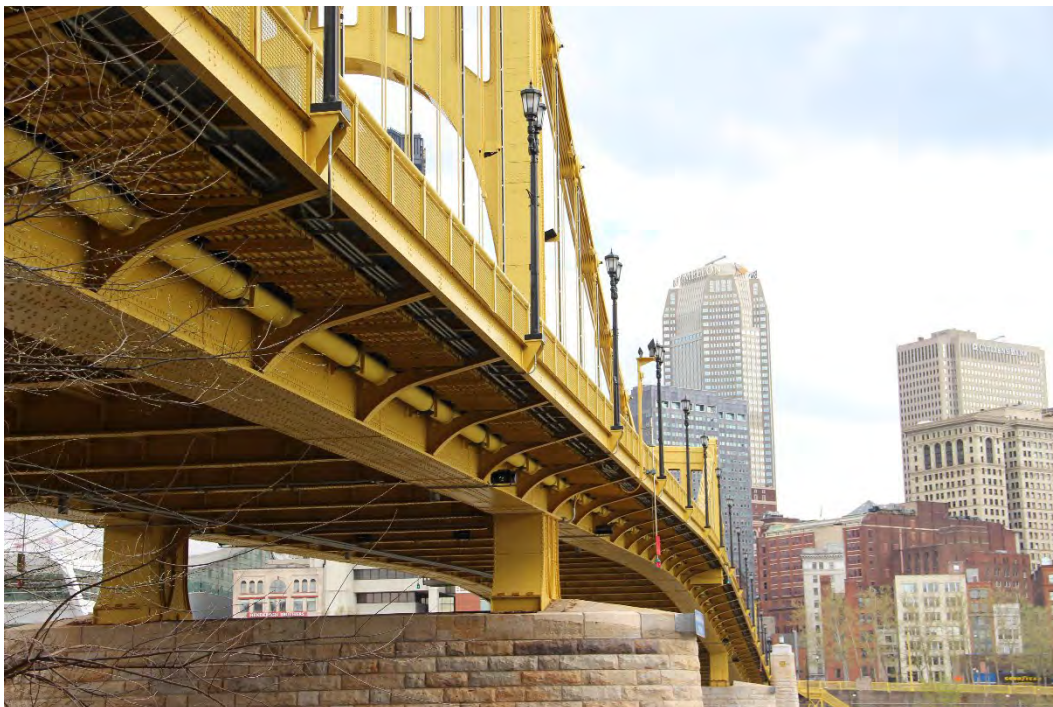
Photo 21. Rachel Carson Bridge (April 2024), overview of underside of west elevation of bridge, facing south from north end of bridge, showing stiffening girder and sidewalk brackets.
