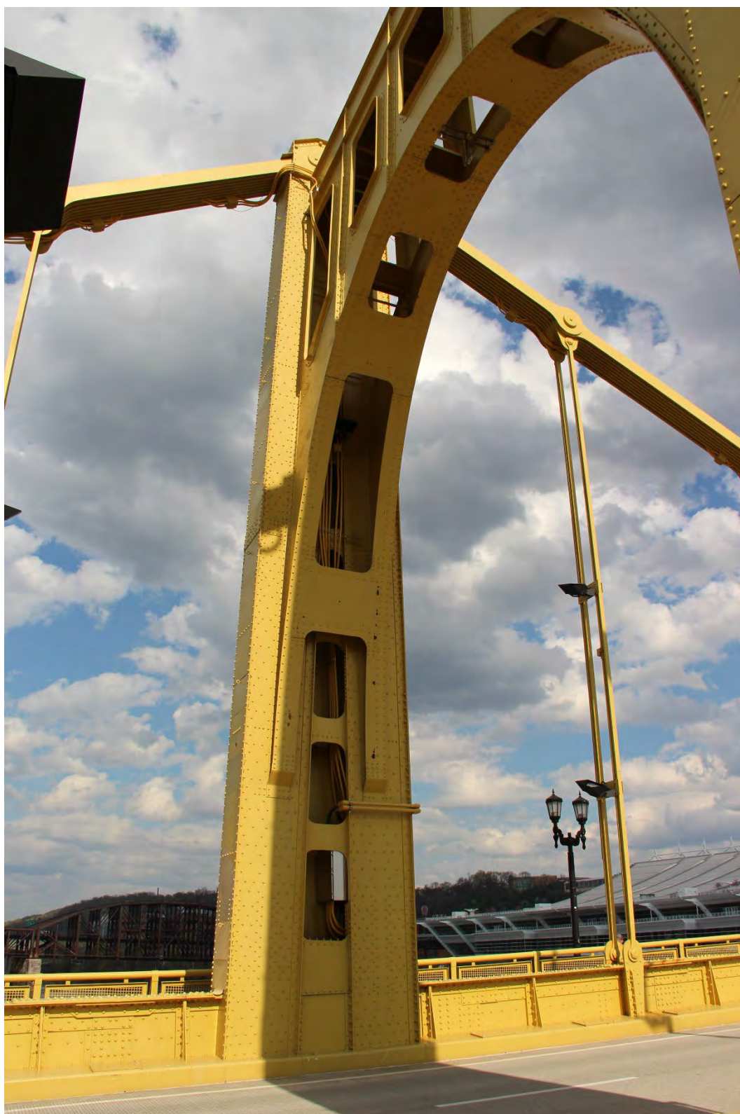
Photo 17. Rachel Carson Bridge (April 2024), detail of arched bracing on north tower, facing southeast.
