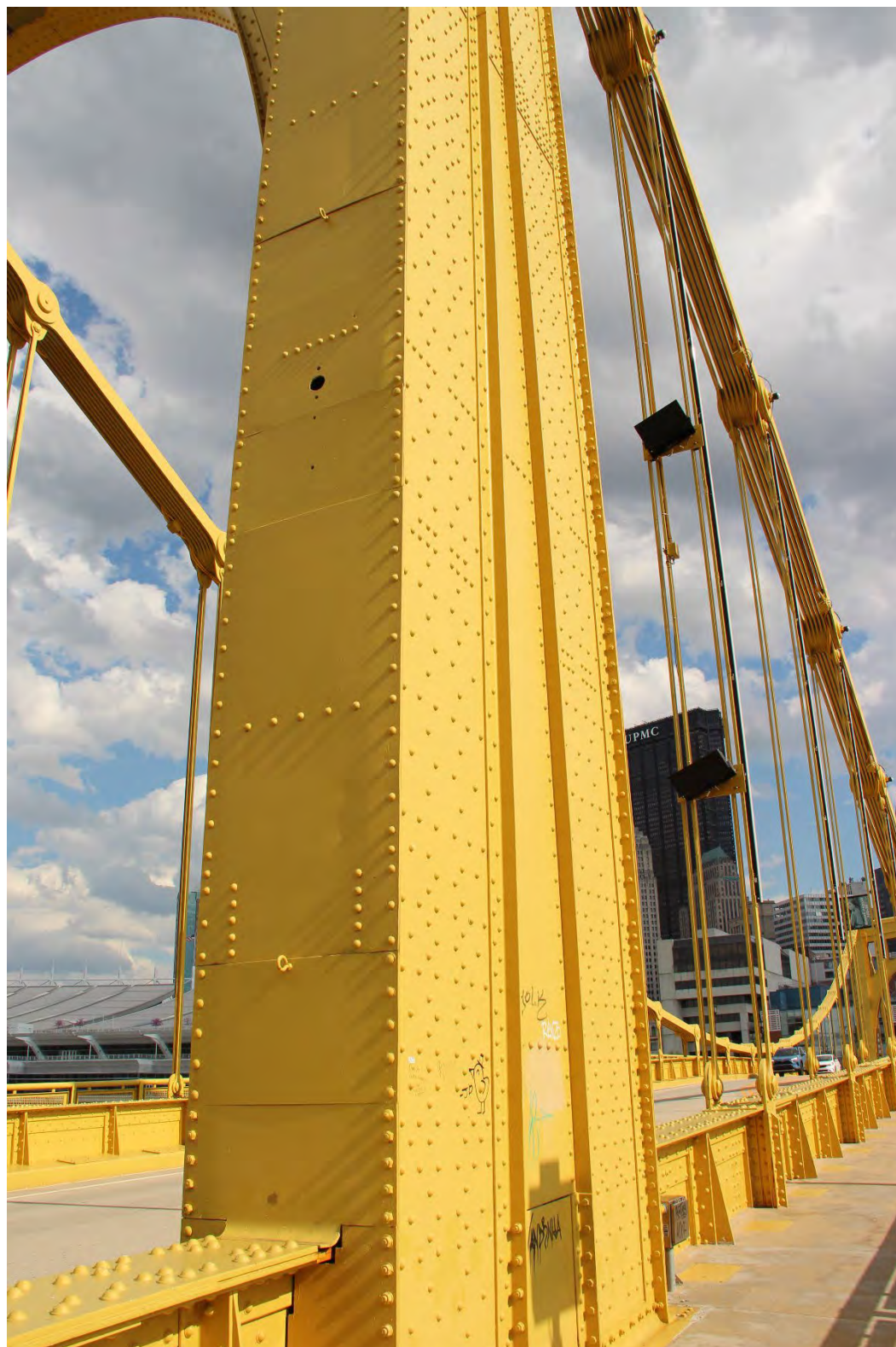
Photo 18. Rachel Carson Bridge (April 2024), detail of north tower showing battered design and built-up, riveted construction, facing southeast.
