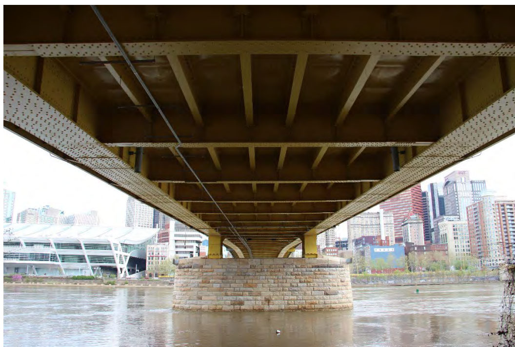
Photo 22. Rachel Carson Bridge (April 2024), underside of north end of bridge, showing stiffening girders, floorbeams, and stringers, facing south.
