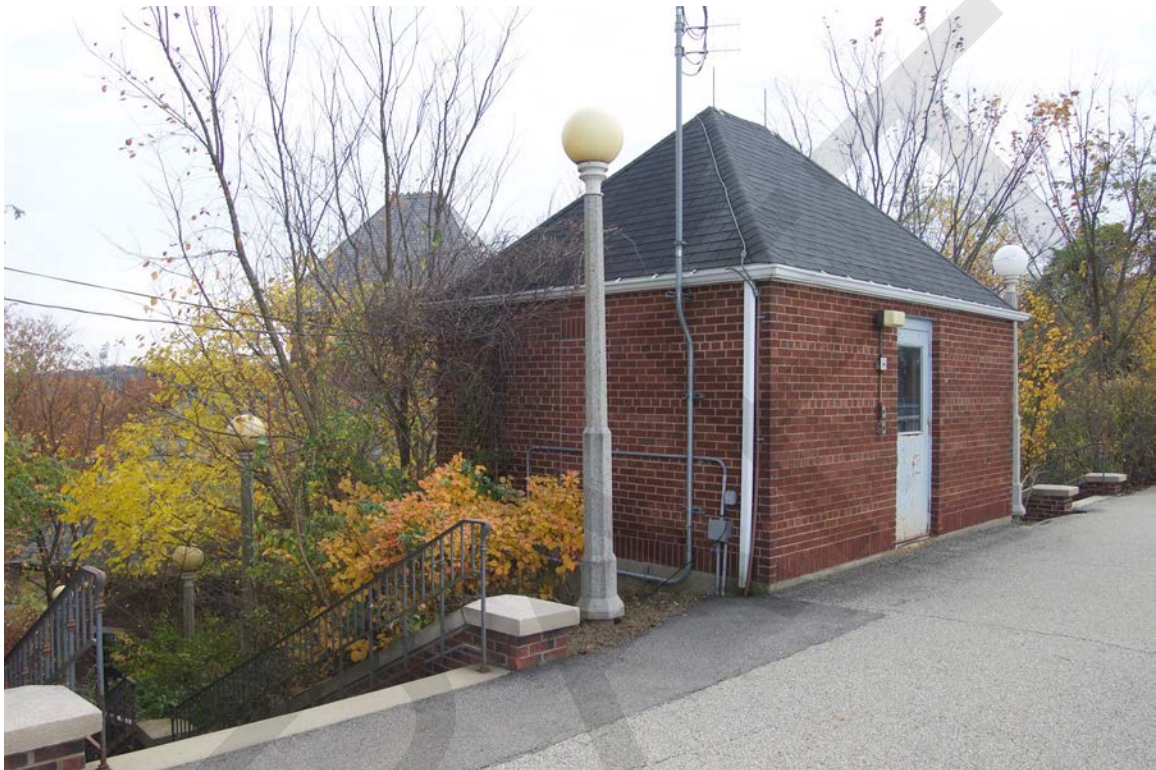
Photo 27. Reservoir service building, Reservoir No. 1
