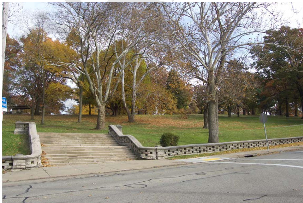
Photo 40. Stone wall and steps, Bunker Hill St.
