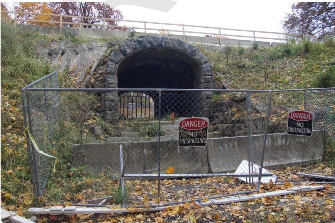
Photo 38. 12' span stone arch carrying Reservoir Drive over Ginkgo Trail
