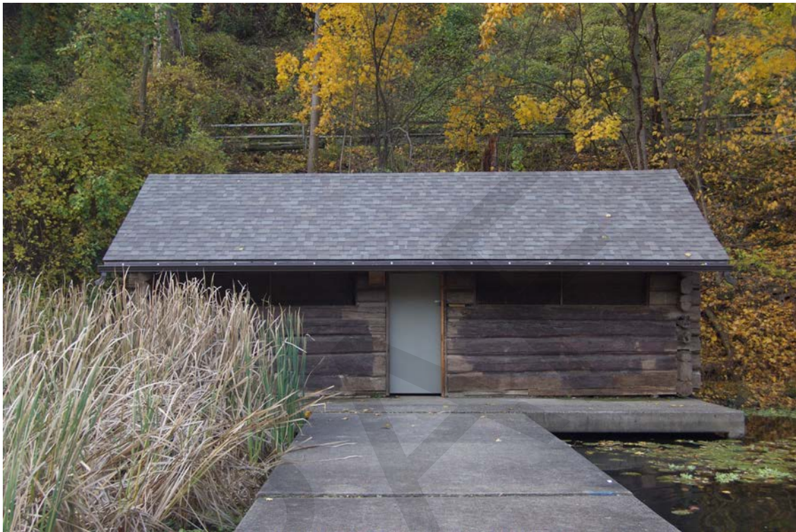
Photo 31. Casting cabin, Lake Carnegie
