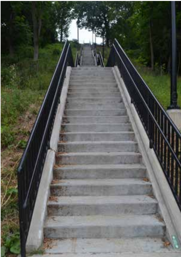
The rebuilt Joncaire Steps include a runnel for bikes and new lighting.
