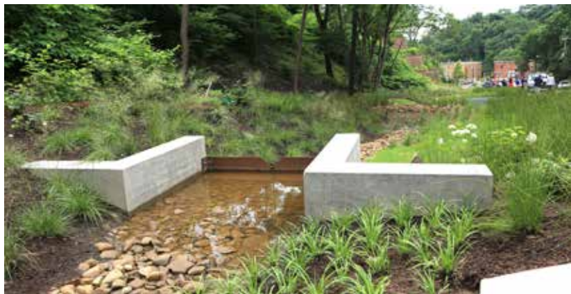
Centre and Herron green infrastructure: Stormwater runoff from surrounding roads is directed into a 585-foot long bioswale that runs alongside the sidewalk of Centre Ave and helps prevent street flooding. Water moves through a series of cascading pools and is absorbed by the ground and plantings. The excess flows into underground storage tanks before being slowly released into the sewer system to reduce overloading of the combined sewer system.
